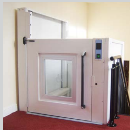
Half Height Gate at Upper Level
